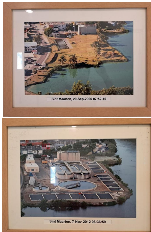
Figure 2-2 – Aerial photos from the WWTP location before and after the first upgrade and enlargement 1
