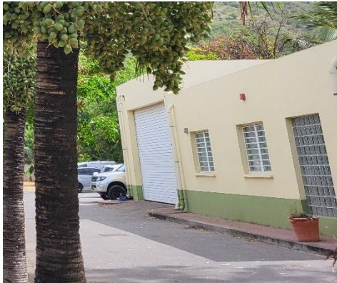
Photo 2-13 - Operation and control building
