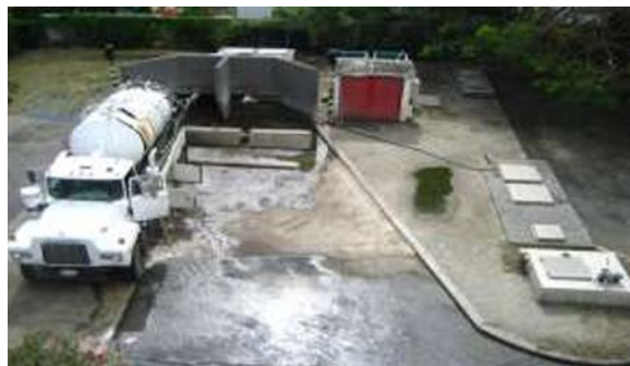
Figure 2-5 – Example of a concrete barrier close to the truck disposal
