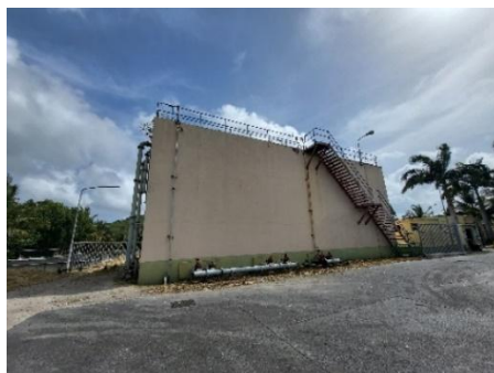
Photo 2-4 – IMHOFF tank building
