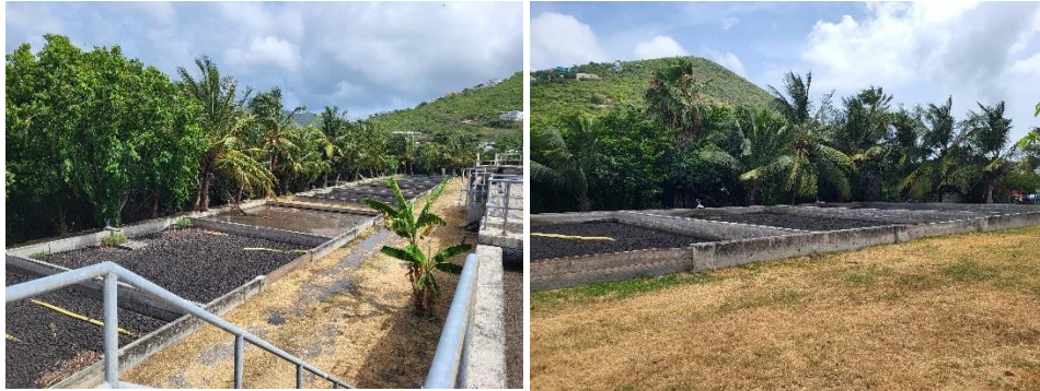
Photo 2-10 – Sludge drying beds (west and north side of the WWTP)
