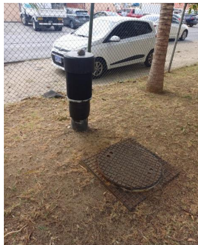
Photo 2-16 – Site of connection with the existing sewage network
