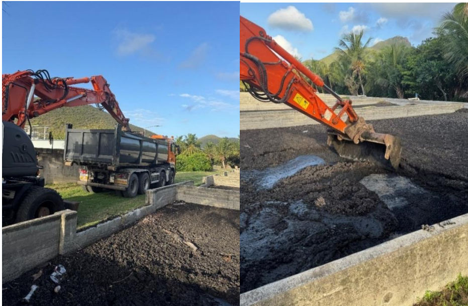
Photo 2-12 – Excavation and transport by trucks (WINKLER, 2025 3 )
