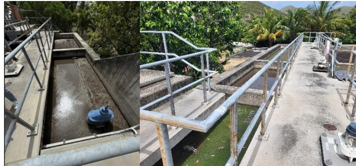
Photo 2-6 – Selector tanks (located at the south limit)
