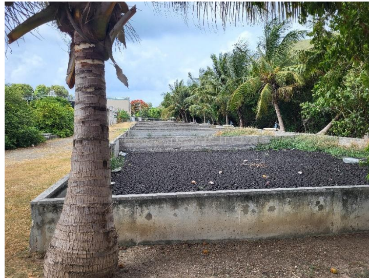
Photo 5-5 –Sludge drying beds (photos from June 2025)
