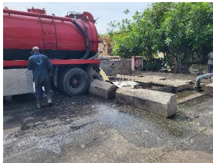
Photo 2-1 - Septage tank discharge sump
