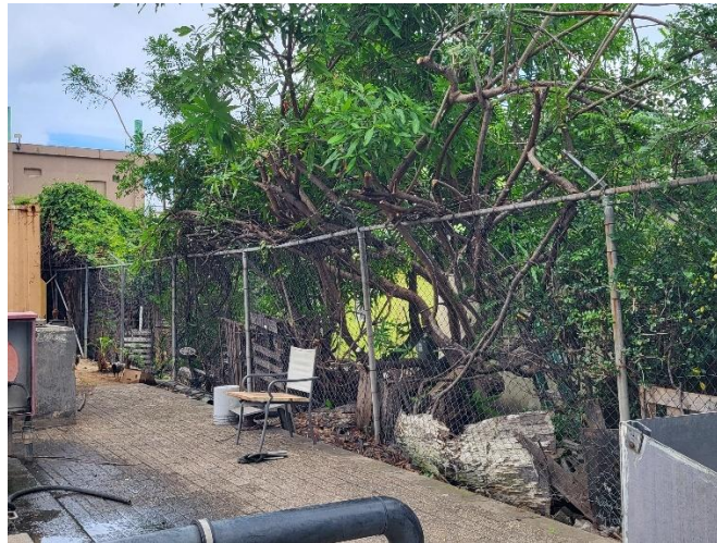
Photo 5-4 –South fence covered with shrubs (photos from October 2025)
