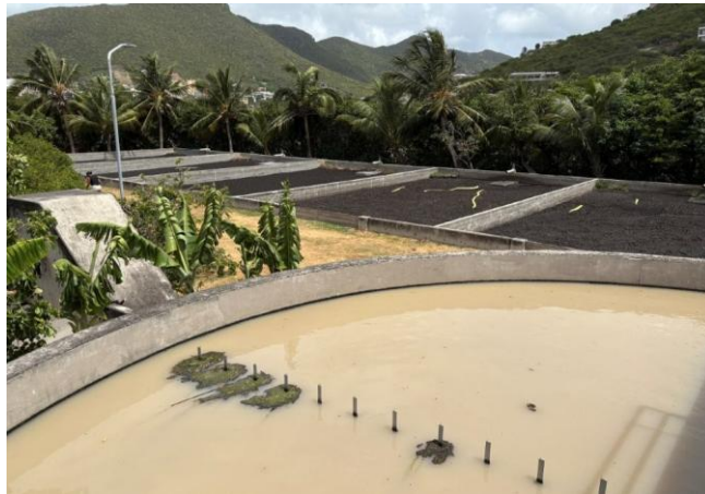
Photo 2-8 – Sludge thickener
