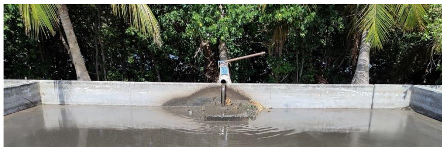
Photo 2-9 – SDB filling procedure (WINKLER, 2025 2 )
