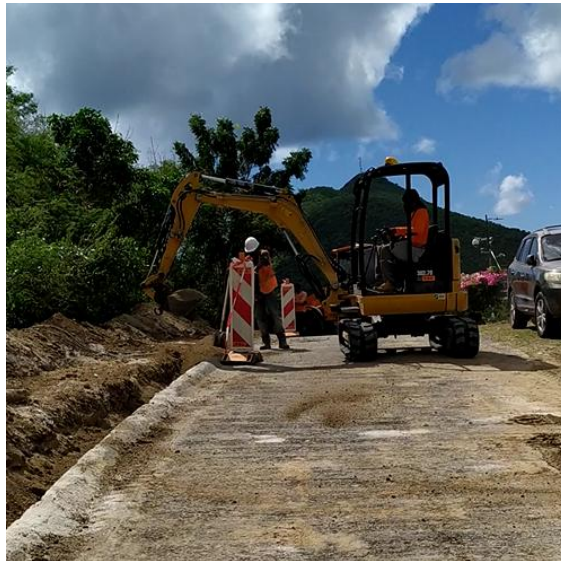
Figure 3: Example of trenching works taking place along a narrow street of Cul de Sac
