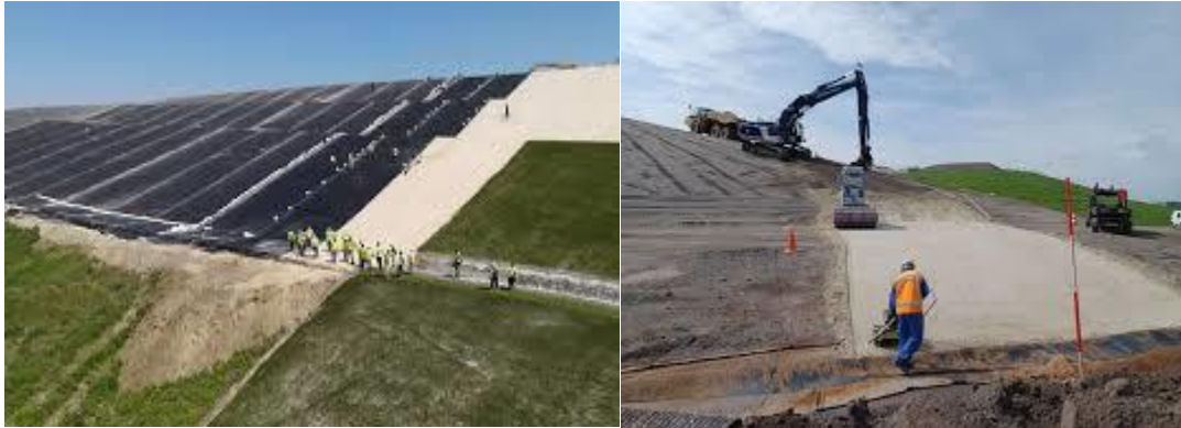
Figure 1.13 Permeability Barrier for Landfill Closure (Synthetic vs Mineral Barriers)
