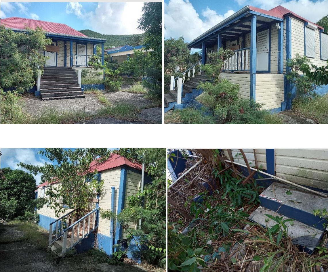
Figure 10. Modern restored Main School Building structure above Feature B; (lower left) new steps on the east side, (lower right) the two new steps at the north side.
