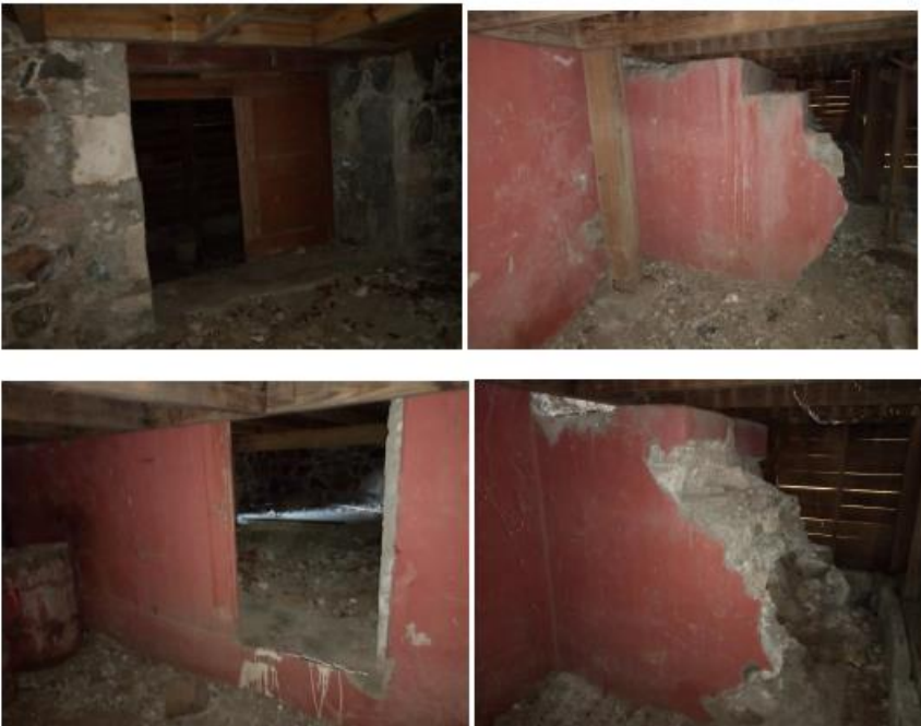
Figure 10. Feature B, Main School Building historical foundations, located beneath the floor beams of the new front porch, with two front steps and a shuttered opening.
