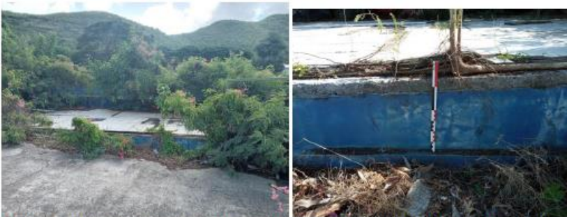
Figure 7. Feature B, being a reduced foundation structure at the CLBS property.
