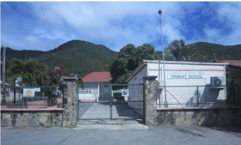
Figure 2. Charles Leopold Bell School, after restoration of Main Building Feature B; and with an expanded large front building, Feature C, present prior to Hurricane Irma.
