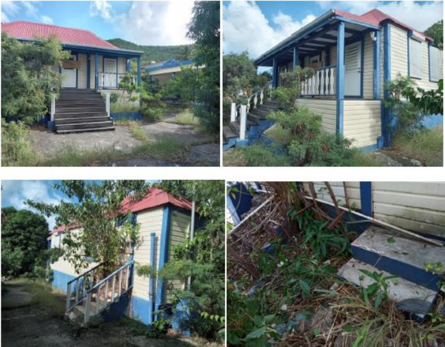
Figure 8. Modern restored Main Building structure above Feature B; (lower left) new steps on the east side, (lower right) the two new steps at the north side.
