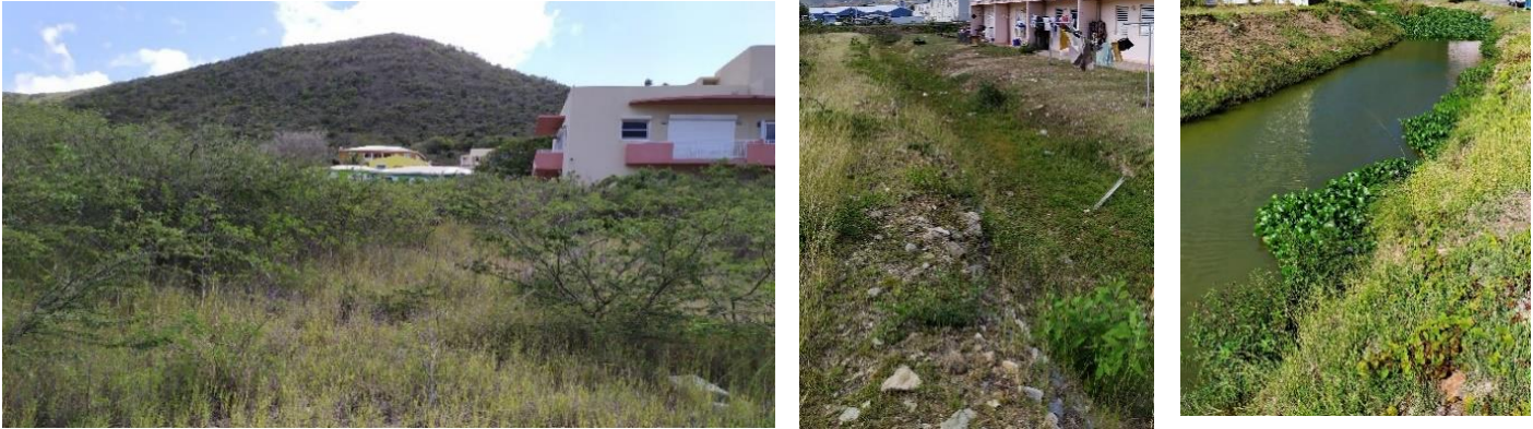
Figure 7: Vegetation overgrowth, draining trench and the Rolandus Canal
