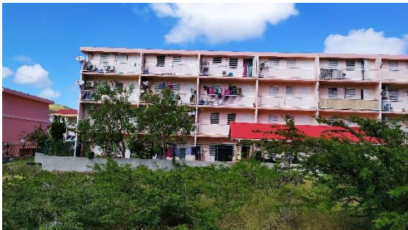
Figure 8: Existing SMHDF houses
