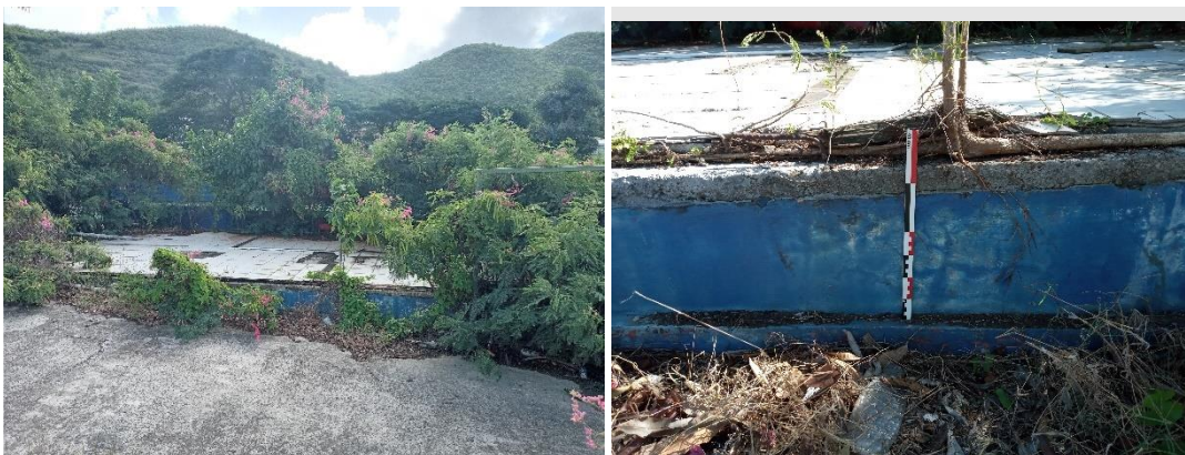
Figure 9. Feature B, being a reduced foundation structure at the CLBS property, these are all that remains of the former police watch-post.
