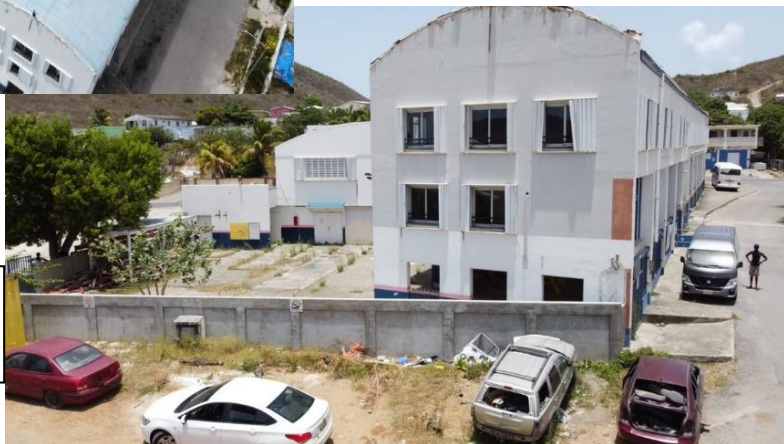
Car wrecks and parked cars around the SML buildings.
