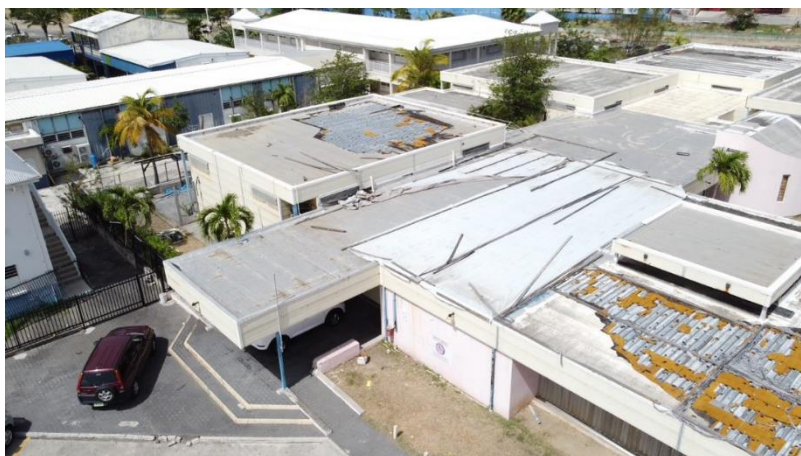
Figure 9: Aerial view of the PJJ
