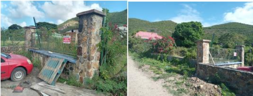
Figure 6. Entrance Gate structure (Feature A) at the CLBS property.
