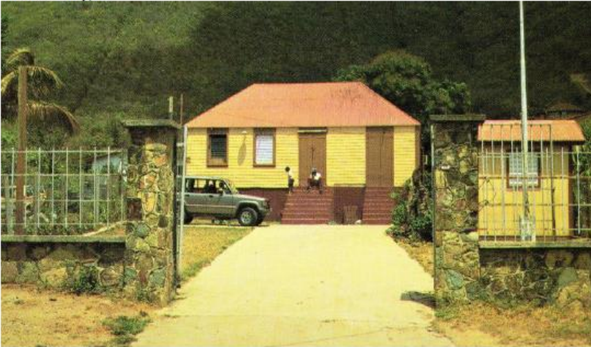
Figure 1. 1970s image of the Charles Leopold Bell School at Cole Bay; (center) Main Building Feature B (note the two front steps and the shuttered opening [behind car] in the foundations); (right) the original small front building Feature C, and (front) the Entrance Gate wall Feature A.
