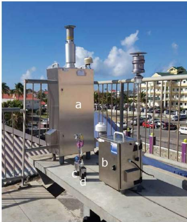
Figure 8 Leckel 24/7 dust sampler (a), KFG dust sampler (b), canister (c) and pump with sorbent tube (d) at the festival terrain (location A)
