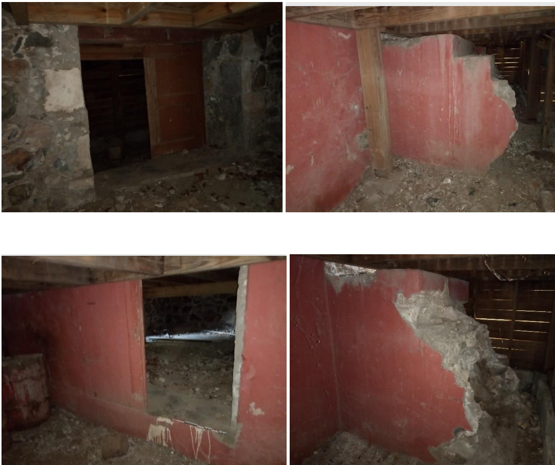
Figure 12. Feature B, Main School Building historical foundations, located beneath the floor beams of the new front porch, with two front steps and an intact shuttered opening.
