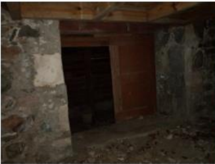
Figure 9. Feature B main building historical sub-floor foundations; (upper left) access opening on the west side; (upper right) interior view; (lower left) north extension discontinuity with older foundation wall, and (lower right) drain opening in north extension, which may indicate it was formerly used as a cistern.
