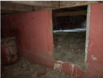
Figure 10. Feature B, Main School Building historical foundations, located beneath the floor beams of the new front porch, with two front steps and a shuttered opening.
