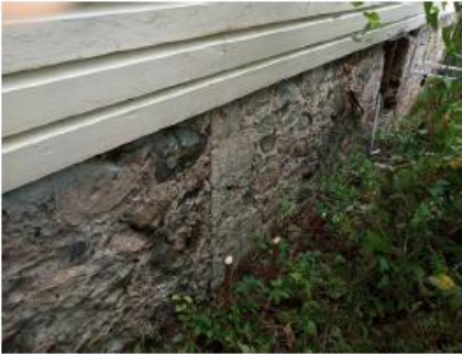
Figure 9. Feature B main building historical sub-floor foundations; (upper left) access opening on the west side; (upper right) interior view; (lower left) north extension discontinuity with older foundation wall, and (lower right) drain opening in north extension, which may indicate it was formerly used as a cistern.
