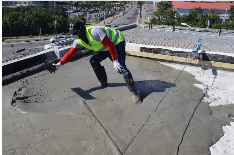
A worker skillfully spreads a layer of concrete on the roof of the Philipsburg Police Station. Repairs works at this station, and the Simpson Bay Police Station, includes making both buildings wind and watertight.
