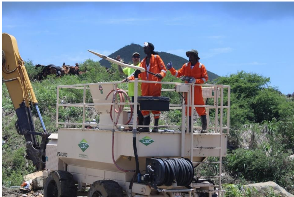
VROMI Ministry workers receive hands-on training on the application of the Alternative Daily Cover (ADC) material. The ADC material greatly reduces the risk of fires and odor nuisances on the landfill.
