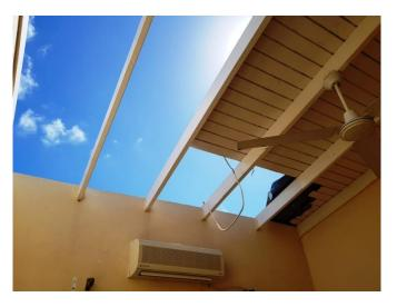
Note the ceiling fan and AC unit that will have to be carefully removed and set aside for re-use by the homeowner.
