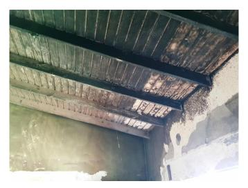
While the damage here is from a storm related electrical fire, the damage is to the roof joists and boarding which will require replacement and are covered under the programme.
