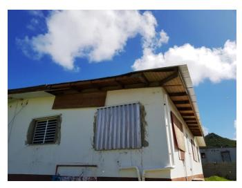
The repaired portion of the roof is without a soffit. In this instance, we would suggest that the new roof incorporate a soffit to match the original as far as possible.
