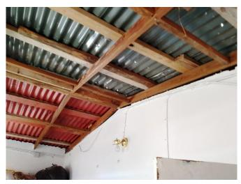
Note the existing electrical wiring that will have to be isolated, removed and then restored.
