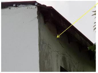
While the homeowner has attempted their own repairs including repainting, the unpainted wall to the right shows what appear to be signs of structural distress. These should either be investigated and specific remedial works included in the BoQ or a Client's Provisional Sum be included in the BoQ.
