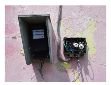
An electrical mains connection that has to be isolated and disconnected prior to the commencement of works.
